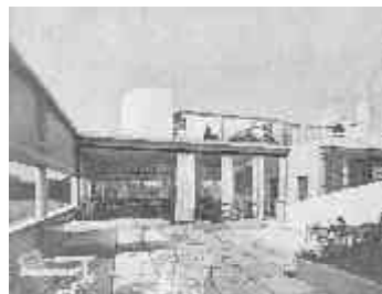
Fig 8.11 - Villa Savoye, roof garden (from Oeuvre Complete )
