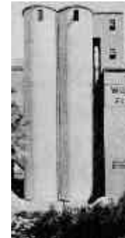
Fig 3.01 - Grain elevator. Primary cylinders - sculpted shade and shadow. ( Vers une architecture )
