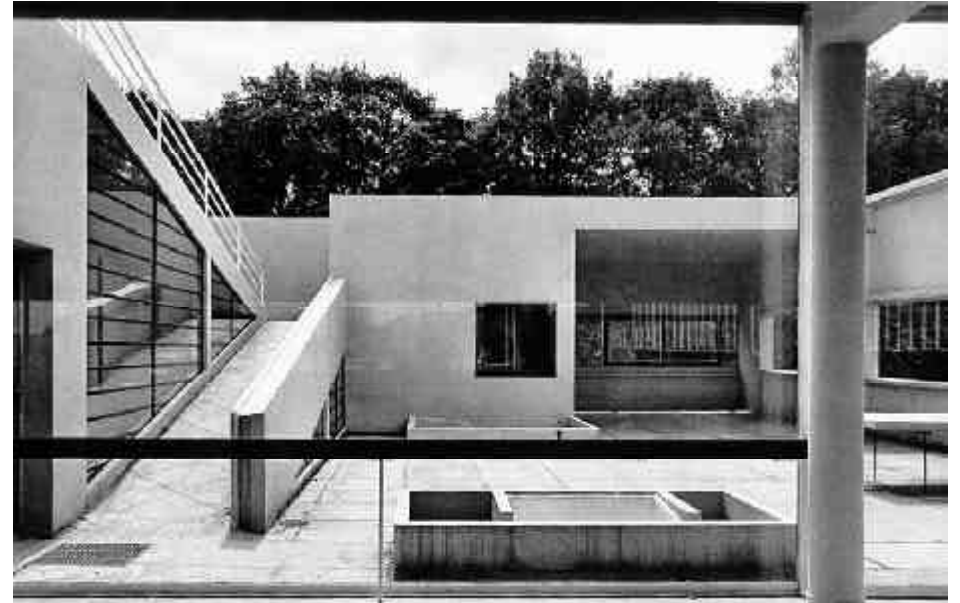
Fig 8.06 - Villa Savoye roof garden viewed from Living Room
