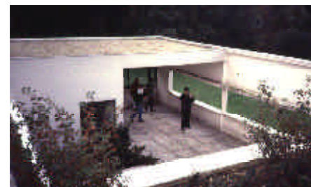
Fig 9.05 - Villa Savoye roof garden
