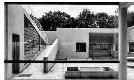
Fig 11.07 - Villa Savoye roof garden
