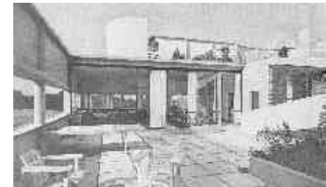
Fig 9.19 - Villa Savoye roof garden (from Oeuvre Complete )
