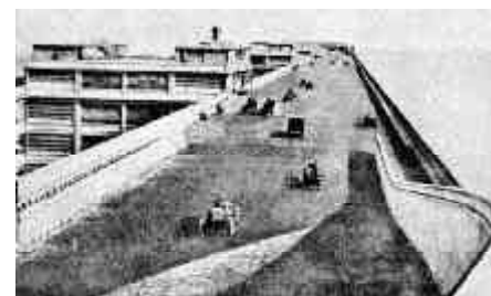
Fig 9.04 - Roof track at Fiat factory, Turin (from Vers une architecture )
