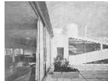
Fig 6.02 - Villa Savoye roof garden (from Oeuvre Complete )
